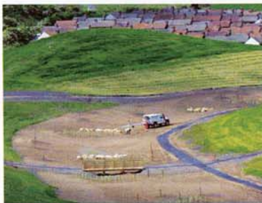
Dalton Park: work gets going on the site
