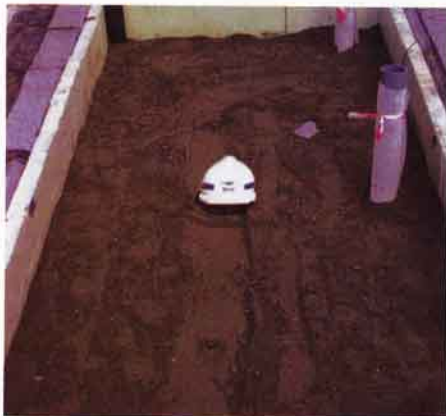
The tree pit soiled and compacted, with cables attached to tree anchors prior to planting.
