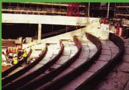
Above: the central arena under construction, summer 2002. Below left: lawn terraces under construction with waterproof layer laid and awaiting installation of the insulation blocks. Below right: the completed lawn terraces in November 2002
