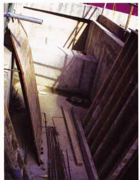
Tree pit detail and tree pit under construction at Paddington Central
