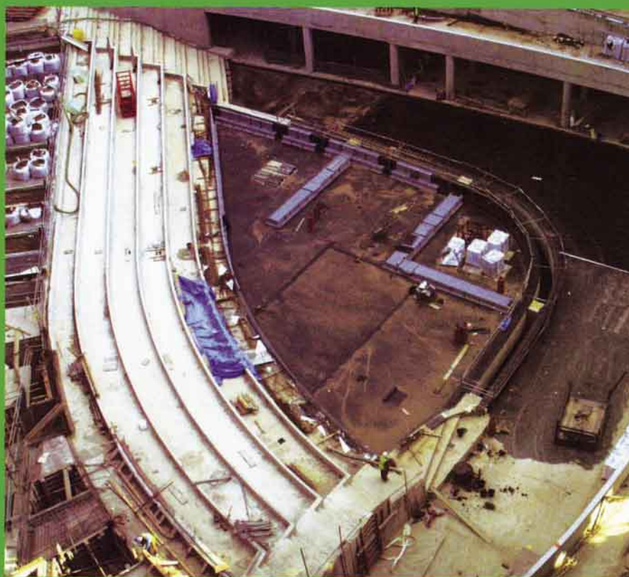
Above: the central arena under construction, summer 2002. Below left: lawn terraces under construction with waterproof layer laid and awaiting installation of the insulation blocks. Below right: the completed lawn terraces in November 2002
